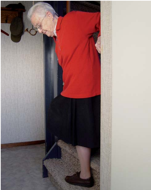
An example of a stair rail that is inadequate to its purpose (photo taken from the Stairway Lab research)
