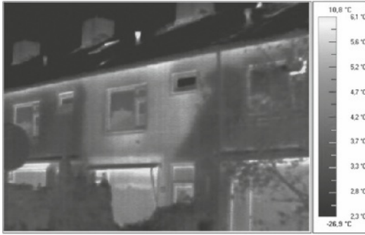
Figure 1.3 Temperature portrayed by an infrared camera
