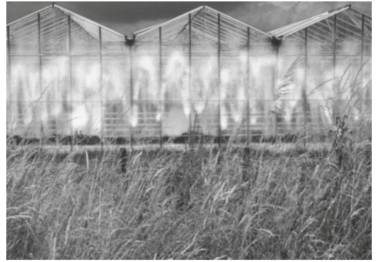
Figure 1.6 White paint preventing overheating
