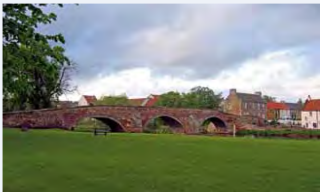
Old Nungate Bridge.
