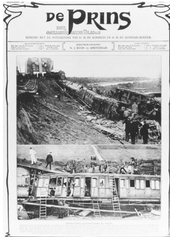
Figure 1-1. Landslide near Weesp, 1918.
