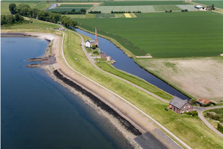
Picture 2.4 The level of the polder lays 4 meters below the level of the river.
