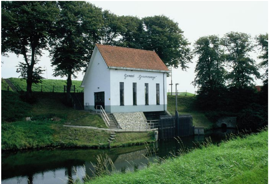
Picture 2.3 Simple pumping station.
