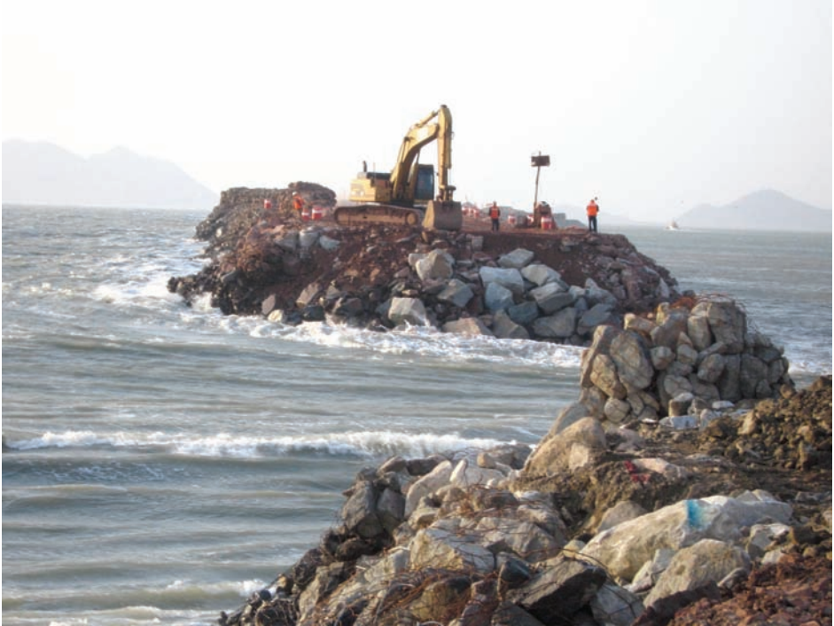
Figure 2-16 Flow in the Saemangeum closure gap just before closure.
