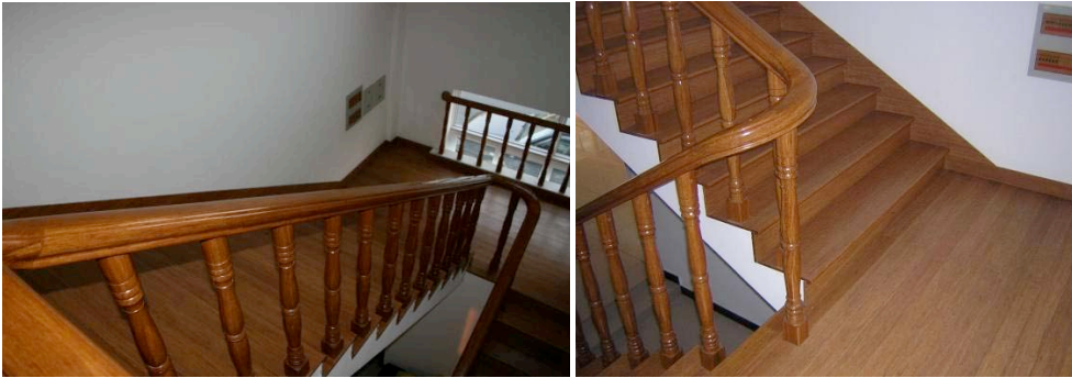
Figure 1.8: Application of SWB in a stairway
