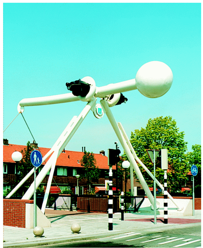
Fig. 1.4 Movable Bridge, Delft
