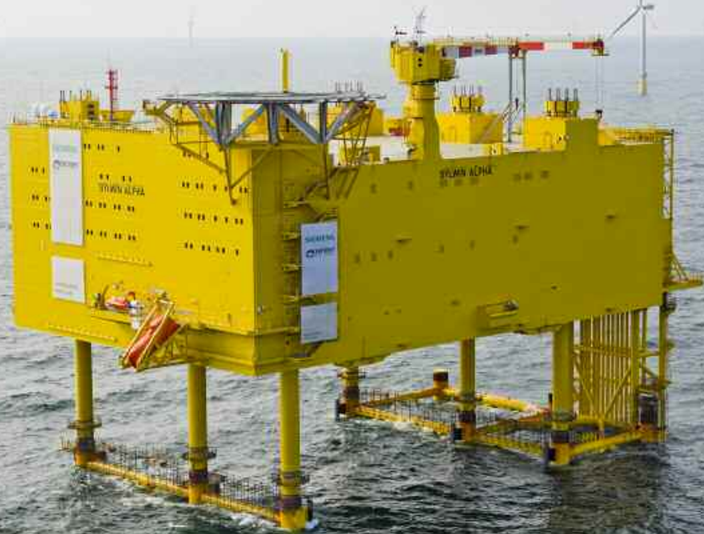
July 31, 2014 – The SylWin alpha HVDC platform, built for Siemens, nearly finished. Engineering company Overdick had conducted the overall design, structural design as well as the transport and installation engineering.
