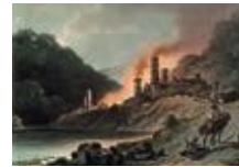
p. 75 Iron Works, Colebrook Dale. R. Bowyer, from a drawing by P.I. de Louthembourg, 1805. Courtesy of and Copyright of the Ironbridge Gorge Museum Trust - the Sir Arthur Elton Collection.
