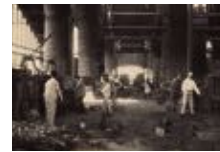
p. 80 Puddling furnaces at Le Creusot, 1899. Courtesy Ecomusée, Le Creusot, France. © CUCM, document Ecomusée. Inv. 2391-4.
