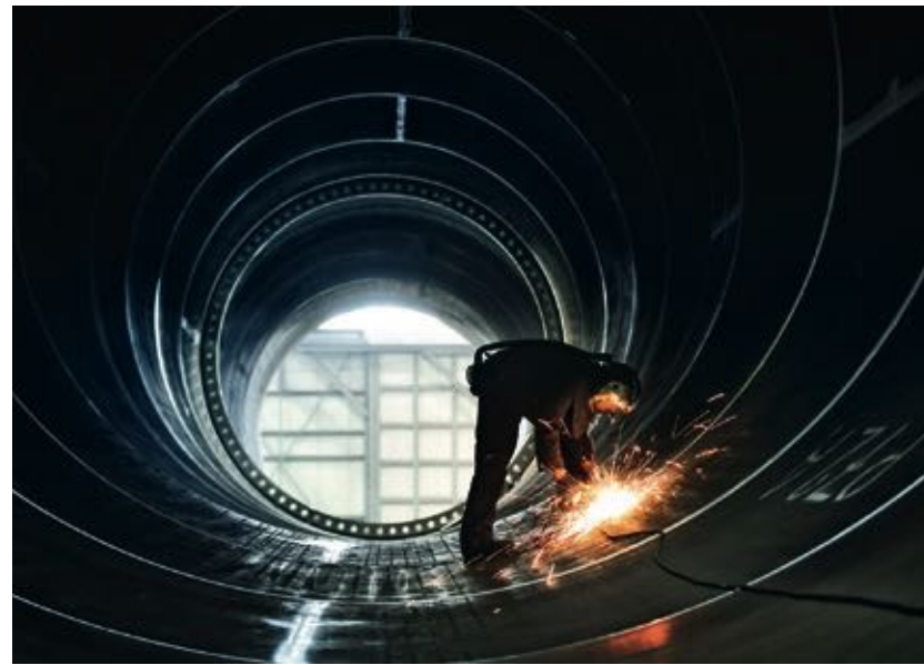
Internal welding of a wind turbine tower
