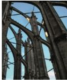
p. 70 Iron rods, Beauvais cathedral. Photo Philippe Dillmann.
