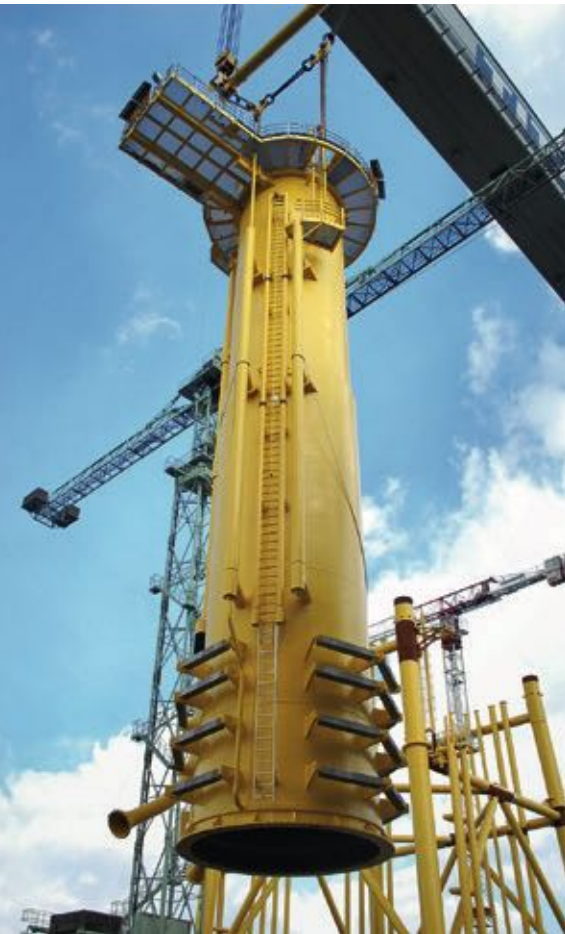
Wind turbine assembly
