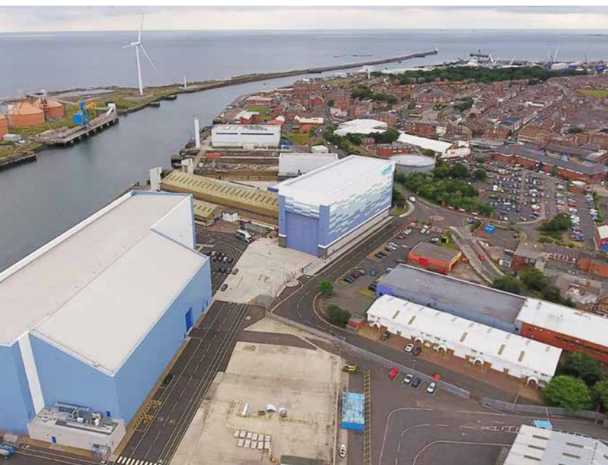
▲ An overview of the test facility complex in Blyth.
