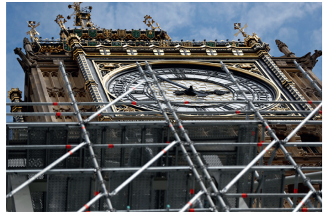
The Big Ben and its scaffolds because it was being restored
