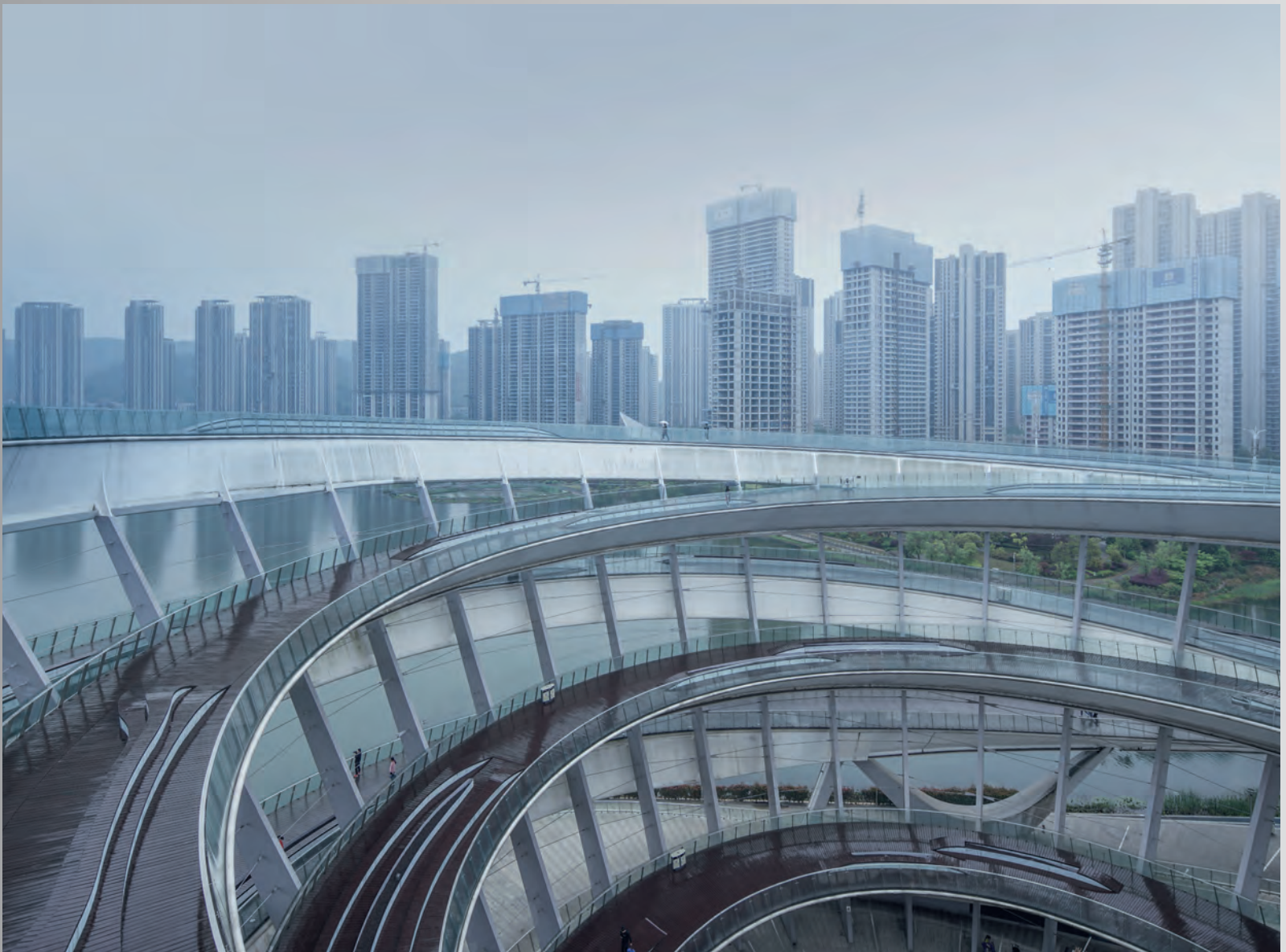
Changsha, Meixi Urban Helix designed by KSP Jürgen Engel Architekten
