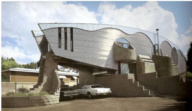
Mead/Rendall Residence, New Mexico, by Bart Prince. Associations with the organic shapes of nature and industrial materials.
