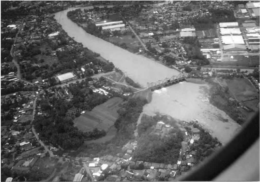
Figure 4: The weir in the Cisadane river (photo WR)
