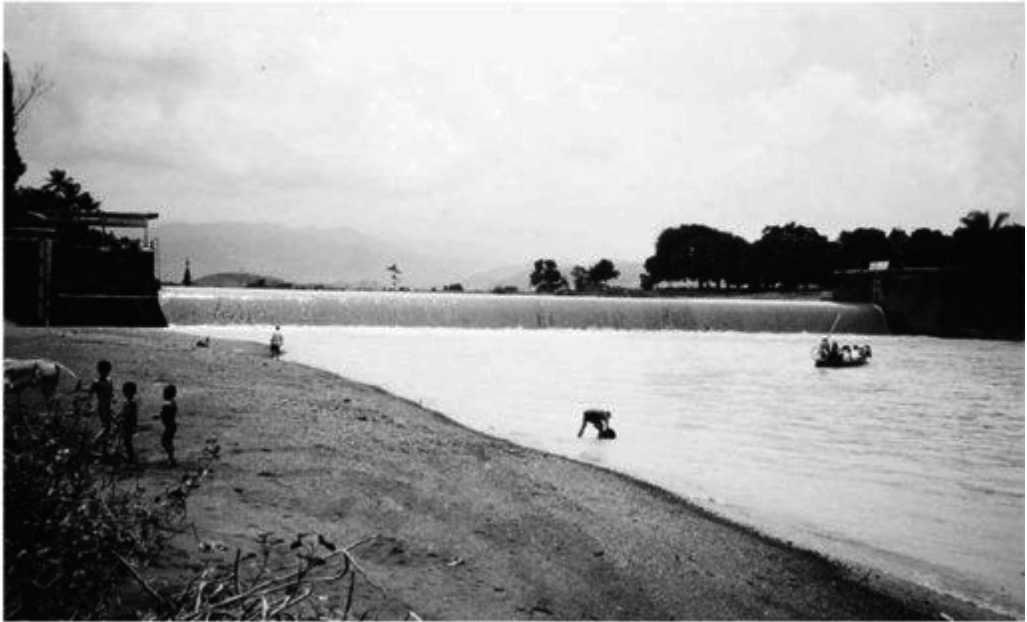
Figure 1: The weir in the Pemali river in the west monsoon period (photo WR)
