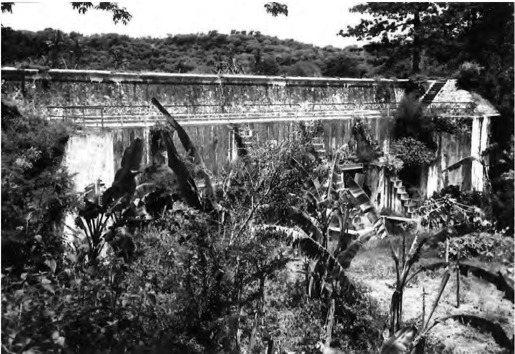
Figure 7: Ruins of irrigation work in the Sampean delta (photo WR)
