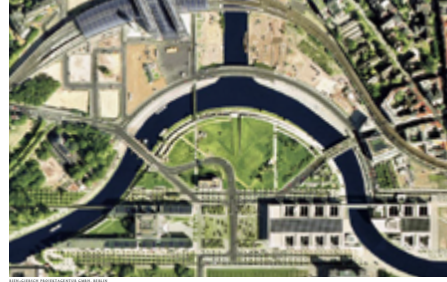
This aerial photograph offers a good overview of Spreebogenpark. In the north the brand new Hauptbahnhof is in the south the strip of government buildings that separate the Spreebogenpark from the Potsdamer Platz. The green space in front of the Reichstag.
