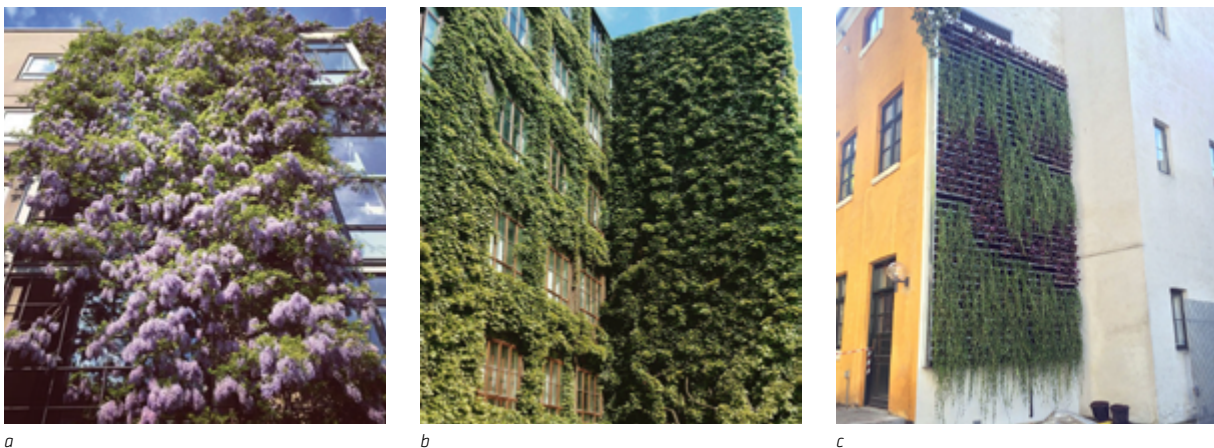
FIGURE 17 Examples of different facade vegetation, showing different colours, shapes, and techniques. The green facades with climbers and creepers are located in Copenhagen (a-b) and the living facade in Aarhus (c). (Images a-b by Ann-Charlott Eriksen; image c retrieved from http://byggros.dk )
