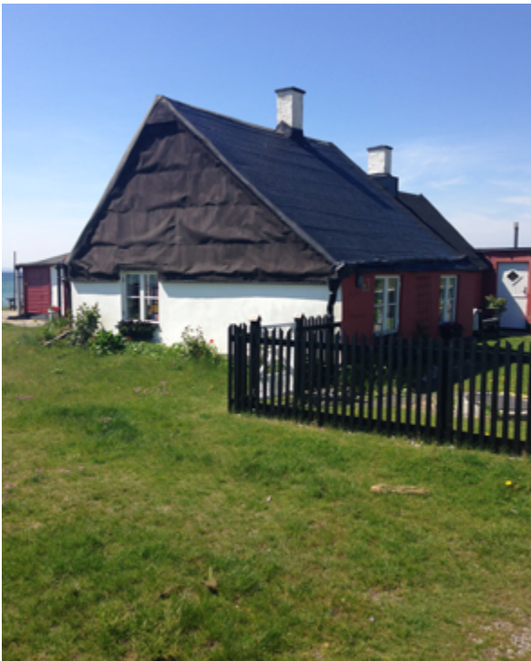
FIGURE 2 Tar paper is utilised for roof and gable cladding at a fisherman's house in Råå.
