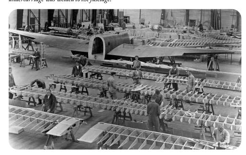
In the front of the picture a pair of lower wings can be seen, with three top wings behind. In the background, Fokker T.V wings are being built, which also included the fuselage centre section.
