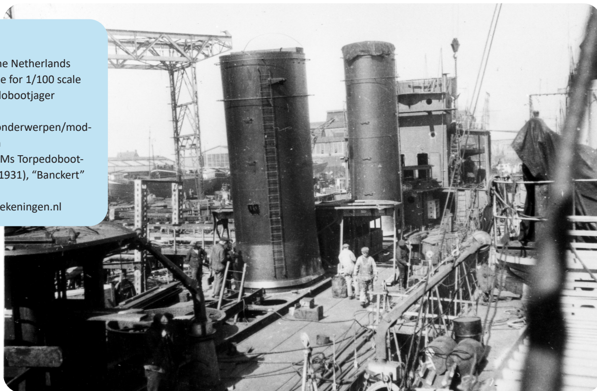
Work on Kortenaer in 1926. The ship would be launched in June 1927.
