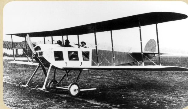
This Wright biplane was flown by T.O.M Sopwith in 1911 during several occasions. This plane was designed by the British Howard Wright and bore no relation at all with the U.S. Wrights Wilbur and Orville!
