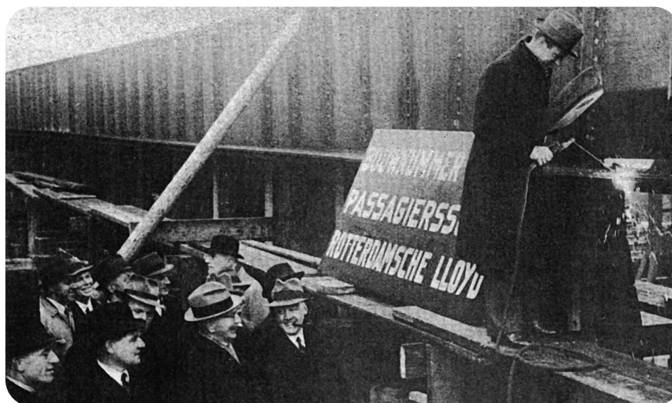
The keel of "Nummer 214", laid down 25 January 1939.
