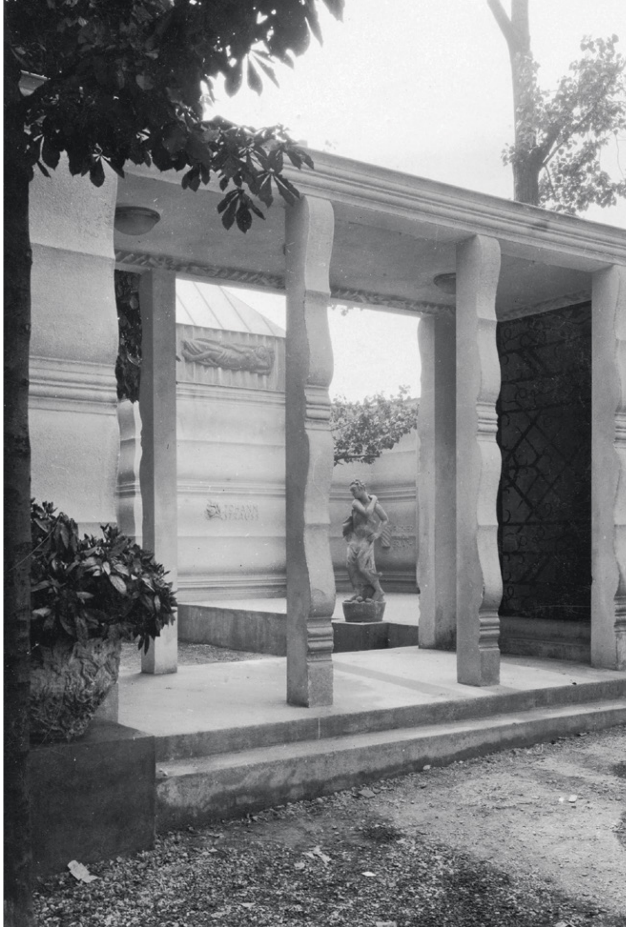
Entrance area and inner courtyard of the Austrian Pavilion at the International Exposition of Modern Decorative and Industrial Arts , Paris, 1925, MAK
