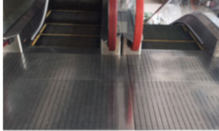
FIGURE 3.8 An example of the VC. The iron platform is a VC connecting the two escalators.
